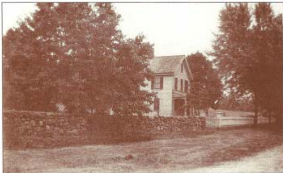
The Follett home and Nursery on Valley Forge Road near the corner of Old Redding Road. 1927
